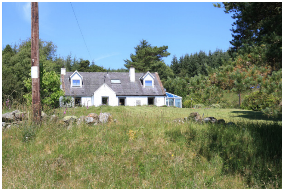
Southern elevation of house and garden area.
